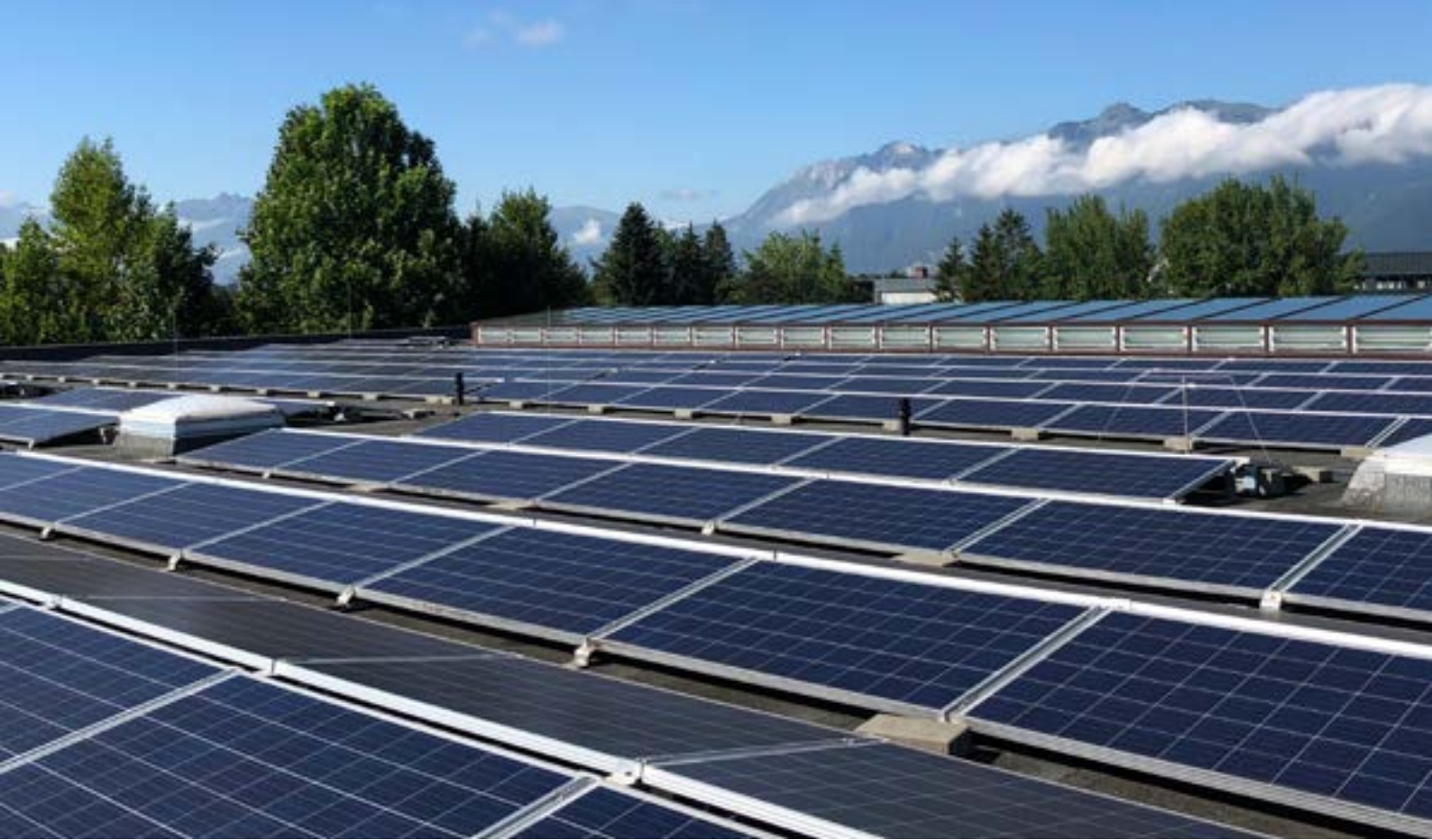
The 360 photovoltaic panels with 93.6 kWp could provide electricity for more than 22 four-person households per year.
