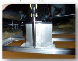
Note: If you need to change the orientation of the image to match the architectural specifications of the room, loosen the Mounting Tabs (C) and rotate the camera assembly as needed. Secure Tabs.
