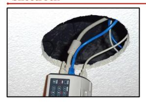
13) Connect all necessary cables to the camera at this time.
