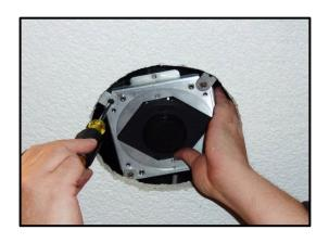
17) Tighten Screws on Mounting Tabs.
