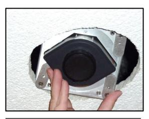
15) Carefully insert assembly with all cables attached into the hole.
