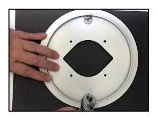
17) Attach alignment ring to face-plate with Nuts (G) provided.
