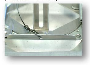
16) Loosen knurled screws and lower camera until flush with bottom of ceiling tile. A straight edge may be used to verify.
