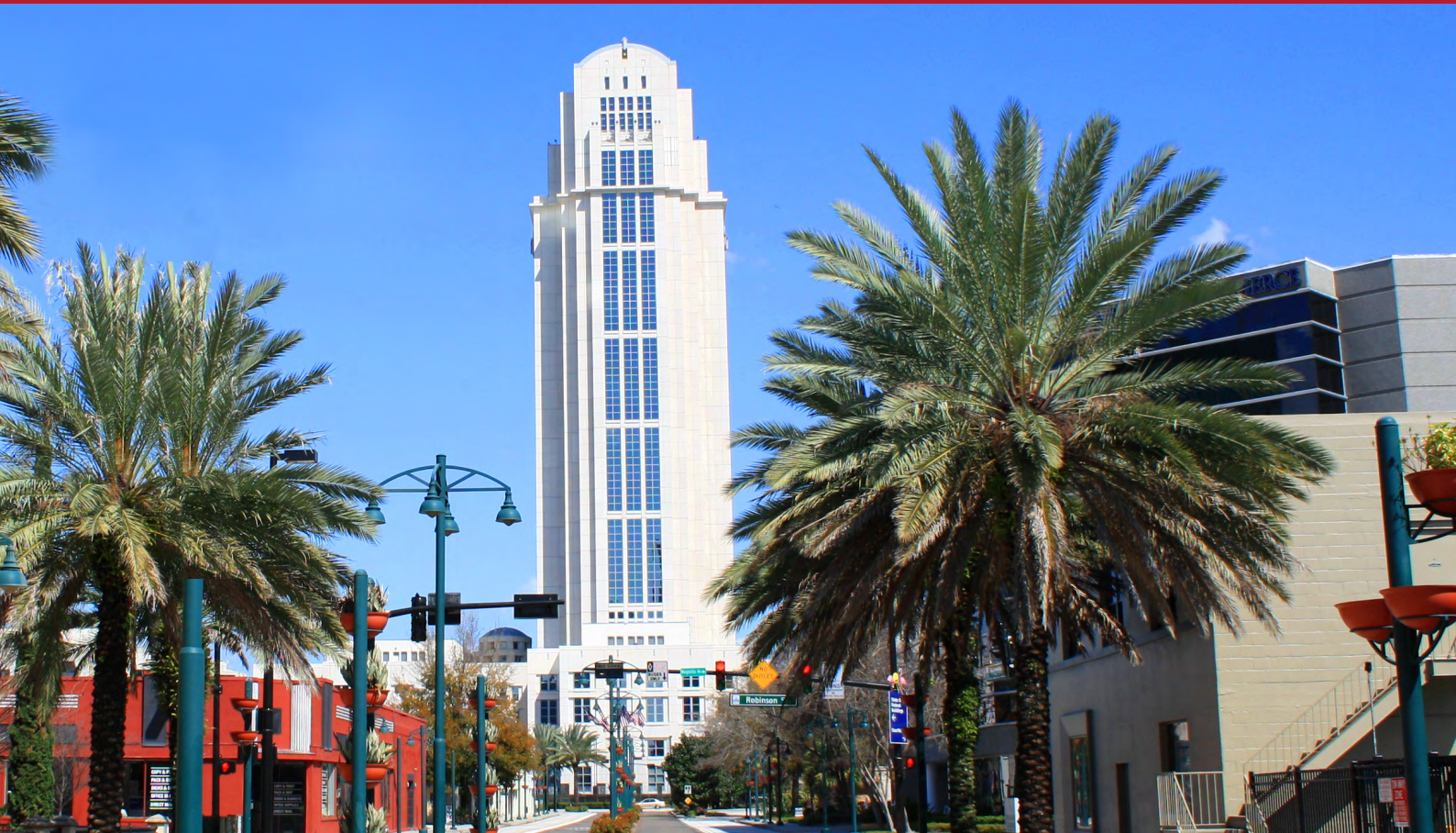
Exterior view: Orange County Courthouse, Orlando, Florida USA
